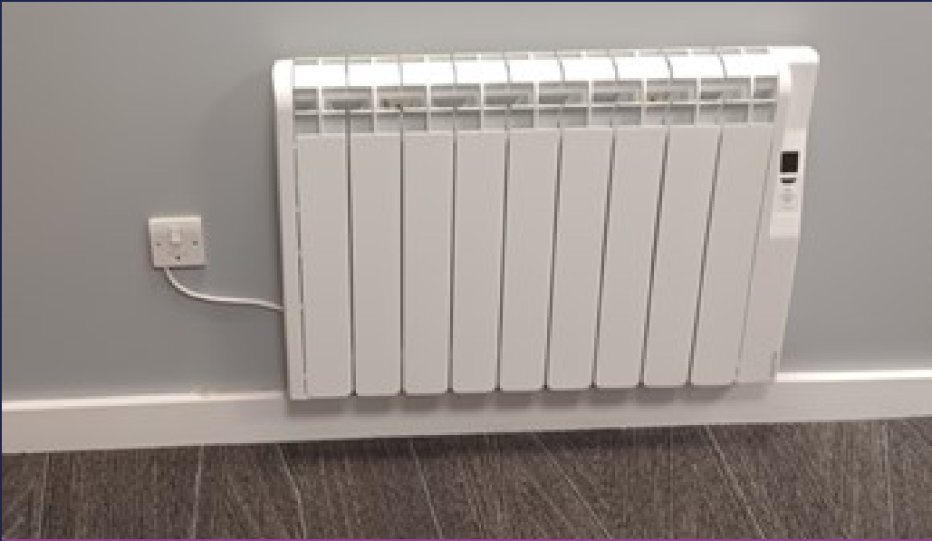
Photo: Wall panel heater replacement
