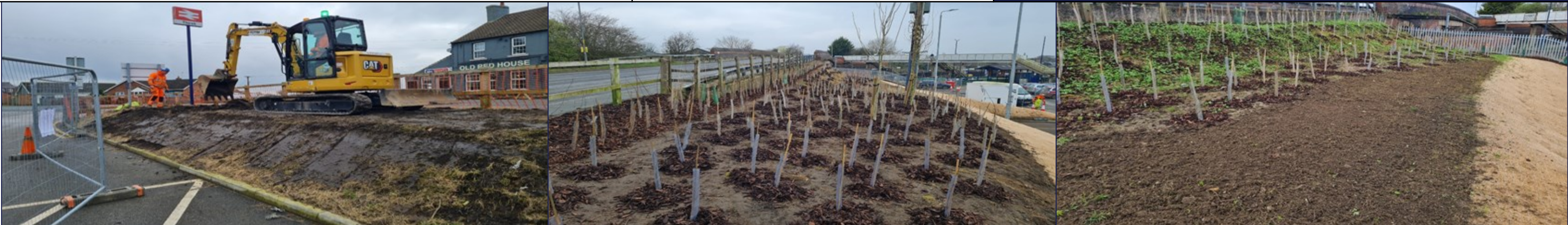
Photos: Thirsk station embankment reprofiling, new scrub and hedgerow planting on the embankment and area prepared for wildflower seed mix.
